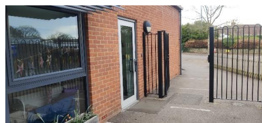
Figure 4.2. Through this gate.
